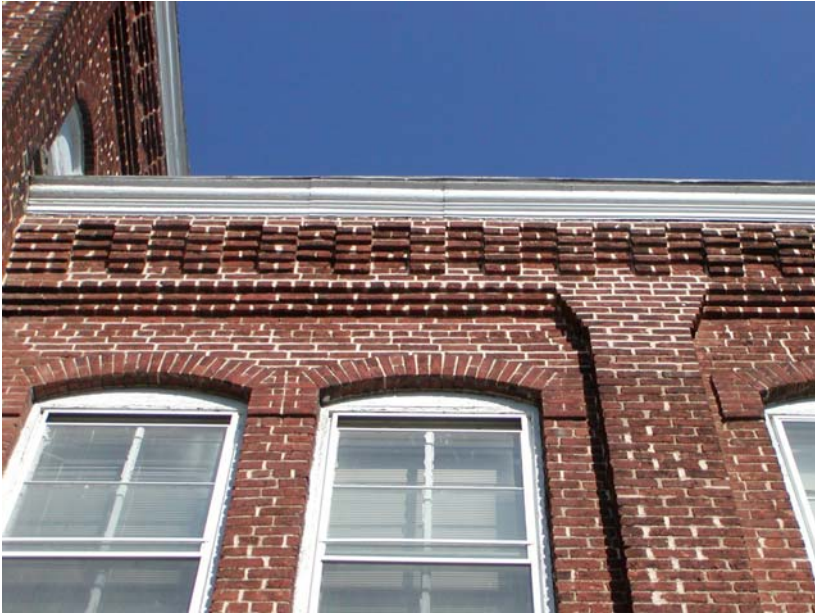
Brick detailing at cornice line
