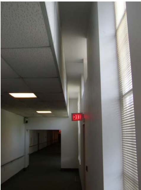
Original ceiling height revealed in corridor
