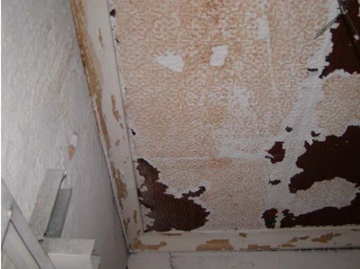
Tin ceiling in corridor
